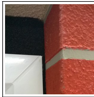
3. Head of frame after settlement - TP450 to head and TP601 to jamb
