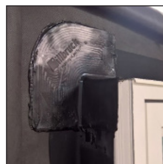
Fig 5: ME241 EPDM Corner applied to projecting window
